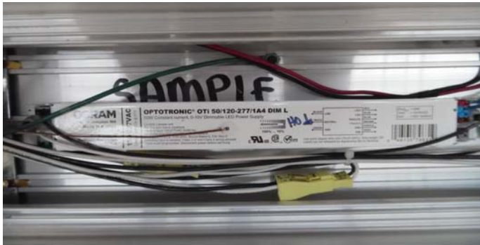
Direct Driver Thermocouple Location
