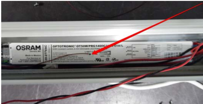
Direct Driver Thermocouple Location
